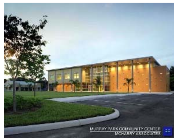
Murray Park Community Center. Exterior photo by Dan Forer.
