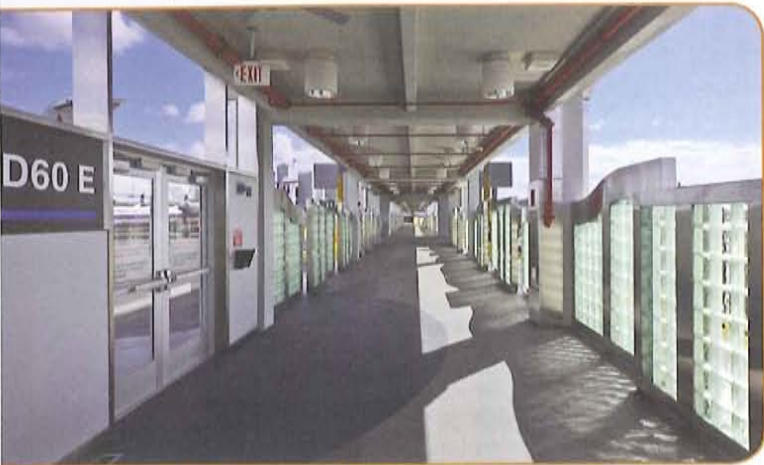
View of regional commuter facility covered walkway, which provides protection from the elements to passengers walking to and from the airplanes.
